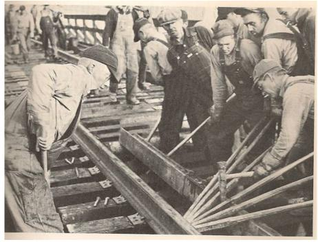
to be cut, and a man struck it one or two blows with a sledge. The rail was then turned over and as many men as could crowd around stuck the end of lining bars under the head of the track rail and bent the rail to be cut down as far as they could.
